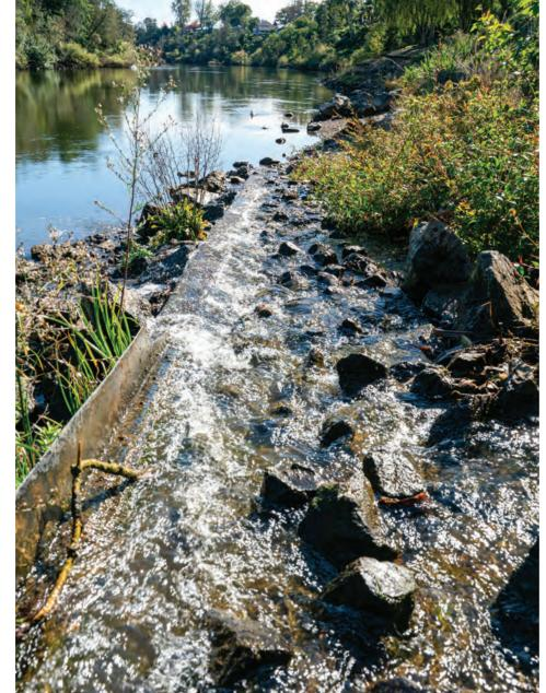
An example of a fish ramp, constructed in 2007, next to the Waikato River. Photo Stuart MacKay/NIWA.
